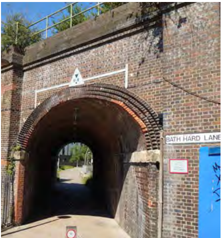
6. Railway underpass opportunity for routefinding
