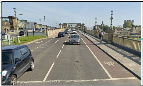
Cycle lane across bridge on southern side of carriageway
