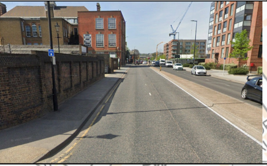
Existing segregated cycle path on southern side of the carriageway
