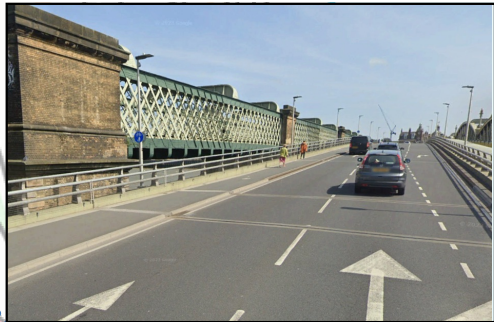
Shared pedestrian/cycle path across bridge on northern side of carriageway
