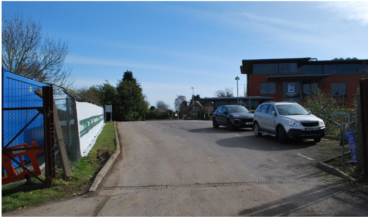
Eastern site entrance to the airport via Innovation Centre and direct link to A229
