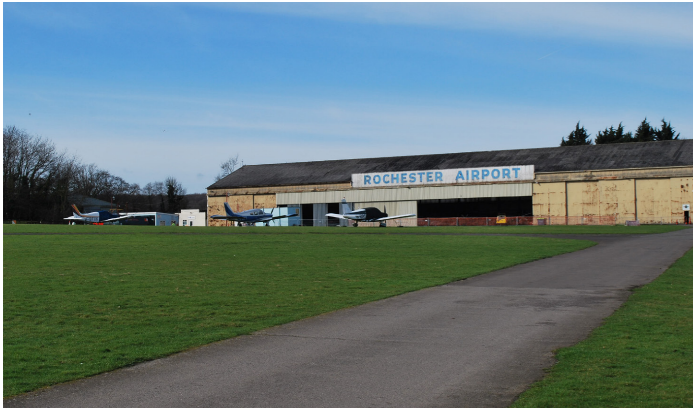
View of existing hangar building on Rochester Airport site
