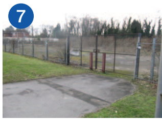
7: Entrance to freehold development land (not used)
